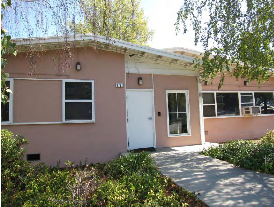
Figure 10. Detail of main entrance of 3701 Hacienda Street, view east.
