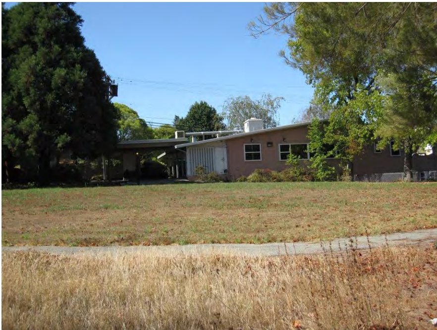
Figure 11. East facade of 3701 Hacienda Street, view west.
