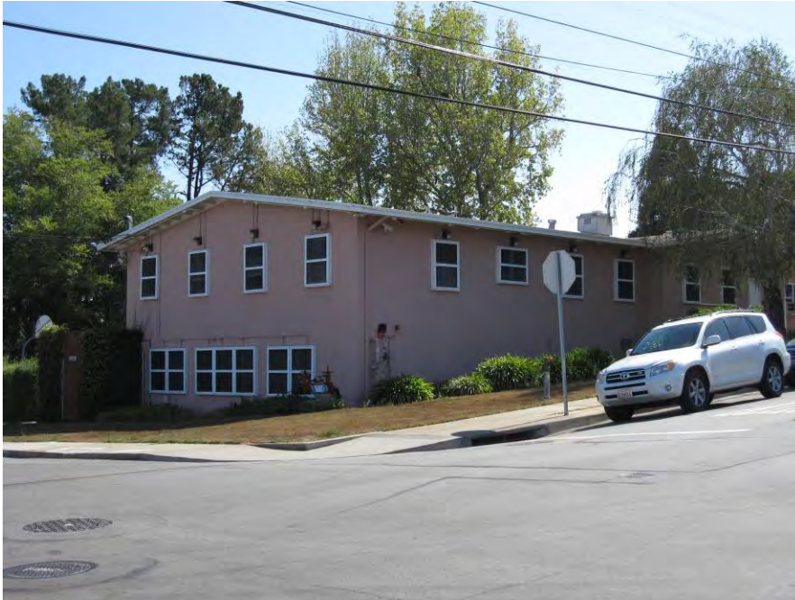
Figure 12. North and west facades of 3701 Hacienda Street, view southeast.
